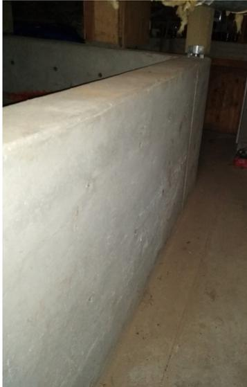
a four-foot concrete retaining wall that rises up to meet the supports under one of the main crossbeams on the southern side. This should create a profoundly more sturdy foothold where once there was only some wood and the notoriously mobile soil of a town built in a river bed. Finally, they replaced the broken supports, and of course mended the exterior masonry where it had crumbled. The cost was \$80,000.
